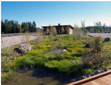
Rain Garden at Parking Lots
